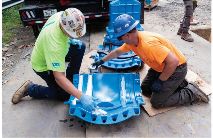
The valve gasket was placed on the pipe to enable its final position to be marked. The pipe was taped, and grease applied to the pipe and gasket which was in place on the valve body.
