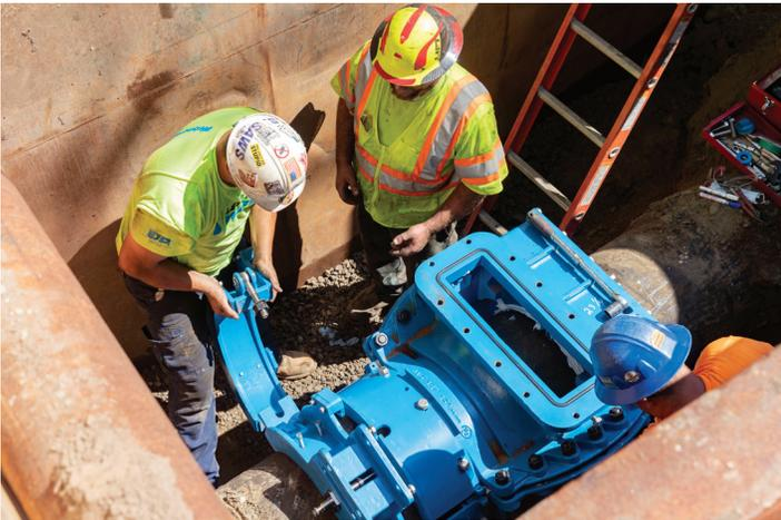
The end rings were installed to hold the gear box.
