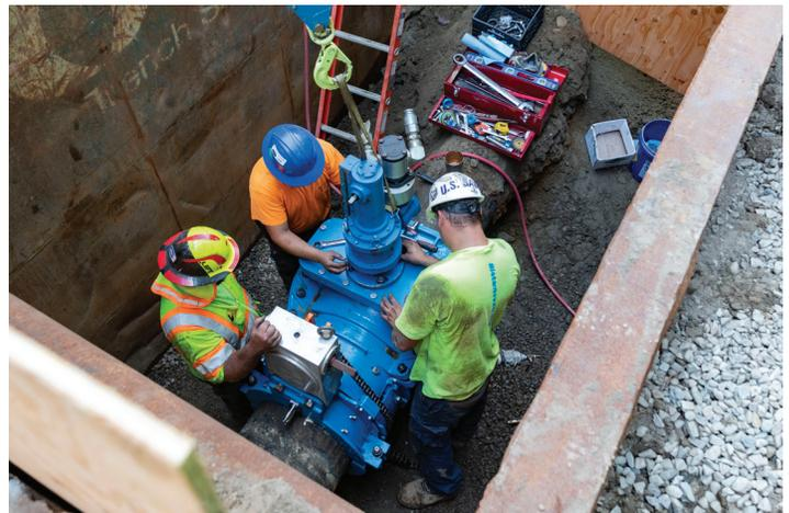
The EM (end milling) machine was installed into the top of the valve.
