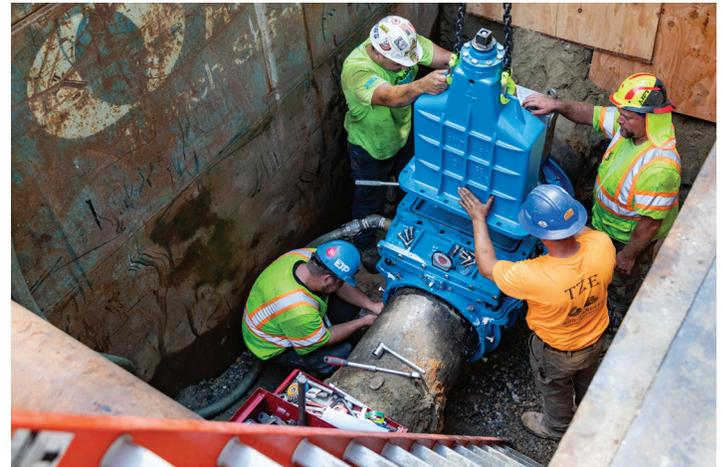
The bonnet wedge was then greased before being lowered into the excavation and fitted to the valve body.
