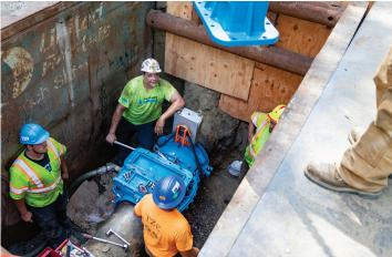
Once connected to the power the EM machine was rotated 120° around the pipe to form a slot which would hold the resilient wedge gate. The isolation gate was closed, and the EM machine removed.
