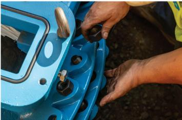
A greased gasket set on the pipe ready to receive the bonnet which was then bolted in place.
