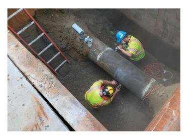
The water line ran under a road which was closed to ensure the safety of the installation crew. The line was then exposed and cleared to enable the smooth installation of the AVT EZ Valve.
