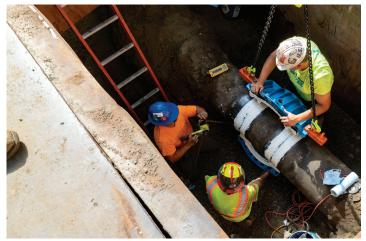
The valve parts were fit together, lowered to the pipe, and set in place.
