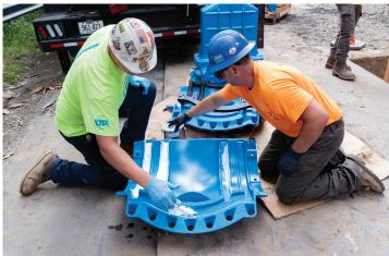
The valve gasket was placed on the pipe to enable its final position to be marked. The pipe was taped, and grease applied to the pipe and gasket which was in place on the valve body.
