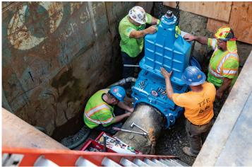
The bonnet wedge was then greased before being lowered into the excavation and fitted to the valve body.
