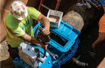
The end rings were installed to hold the gear box.
