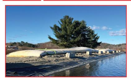
Tim Dagesse, Operator at The Town of Barton Wastewater Treatment Plant, contacted Team EJP South Burlington for sledge bags for a local project. The bags measured 45′ in diameter and 80′ long! Team EJP′s Rob McLaren also distributed knife gate valves and HDPE fittings for the manifold between the bags. P&H Senesac of Milton, VT, did the dredging and pumping into the bags, and J. Hutchins Inc., of Richmond, VT, performed the site work in prep for the bag placement. ■
