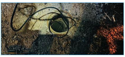
Late one Friday afternoon in April, a client reached out about leak detection services for a project in Dracut, MA. 1,400 feet of 12" lined ductile iron pipe wouldn't hold stable pressure and prolonged the project's completion. Nick Bates, GIS Specialist based out of Gardiner, ME, immediately jumped to get the client the assistance they needed. Nick was on-site by the next night to work with the client to detect and define the problem.
