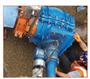
Solution: Team EJP worked alongside AVT to install a 16" EZ Valve so that, should they ever need to, the city may easily shut down the main feed line.
