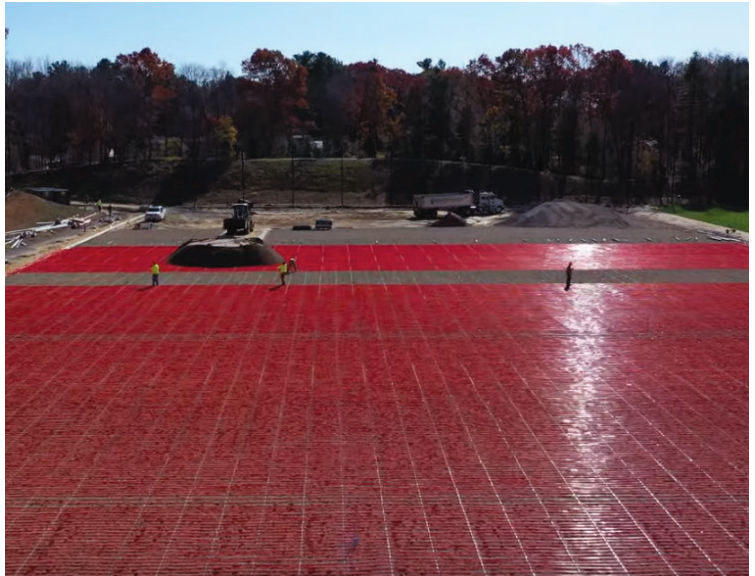
A drone captures an aerial view of the new field construction.
