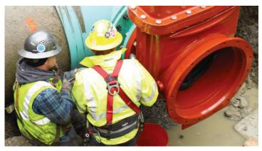
Team EJP's Service Department was recently on the job for Sappi to repair a problem with a 36" Pre-Stressed Concrete Cylinder Pipe. Sappi had noticed a leak beginning to surface on their critical raw water feed line, which feeds their entire property and production facility.
