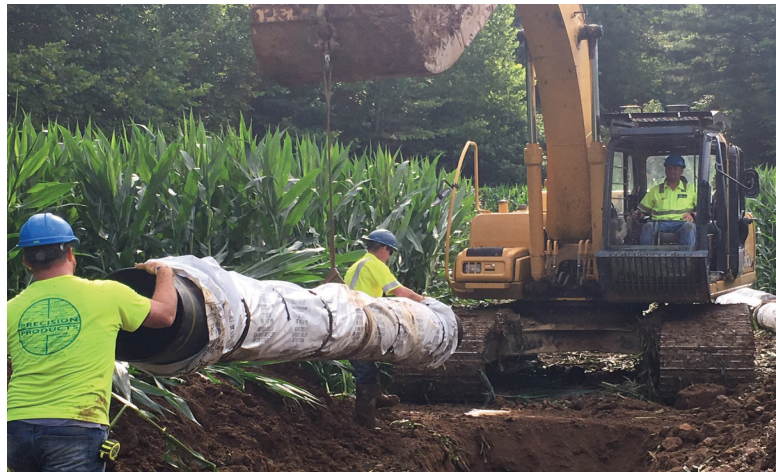
V-Bio poly-wrap on the American Zinc Pipe seen here is added protection to help improve the longevity of the pipe in highly corrosive soils.
