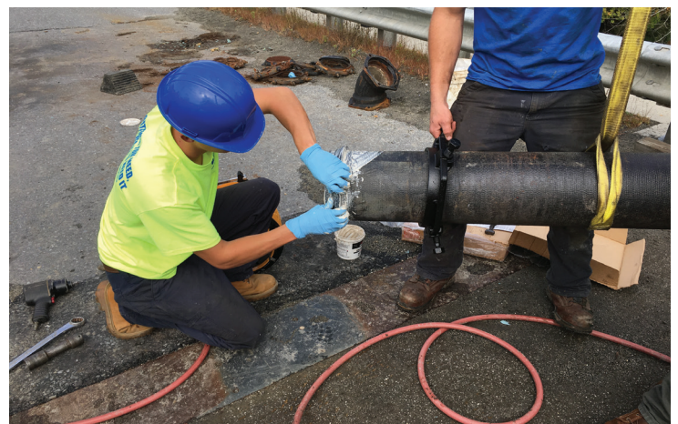
EJP Service Technician Patrick Coughlan is seen here installing a gasket on a piece of ductile iron pipe.
