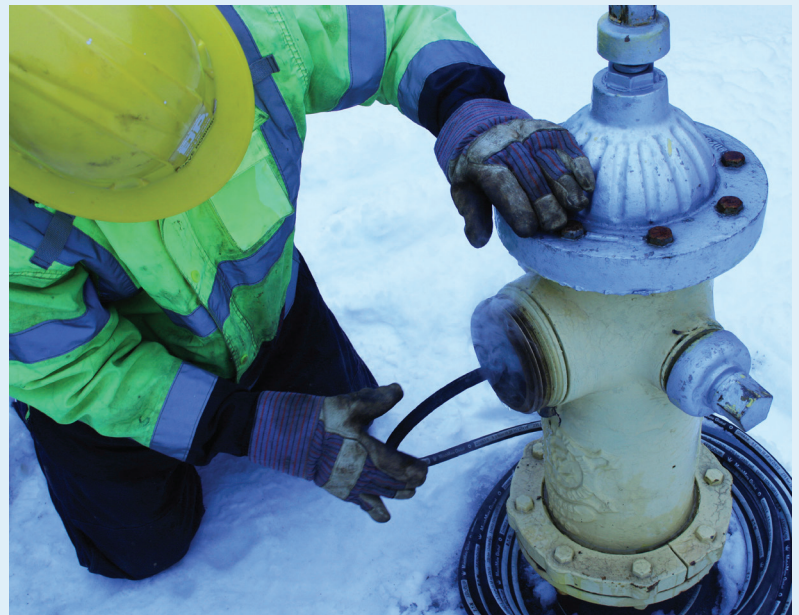
EJP service tech Dave Robinson seen thawing a hydrant
