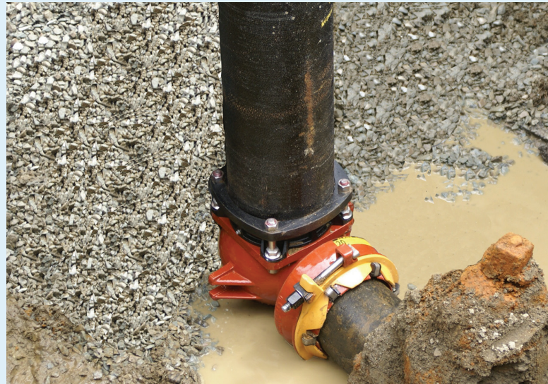
This ALPHA restrained joint easily slips on a pipe in Pittsfield, ME
