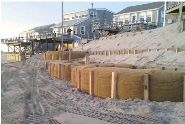
NETCO, a coastal erosion control contractor from Lexington, Massachusetts, utilizes high-density coir fiber matting to fabricate sand-filled coir envelopes to protect coastal property. One of their Rhode Island projects was featured on the PBS television series, "This Old House".
