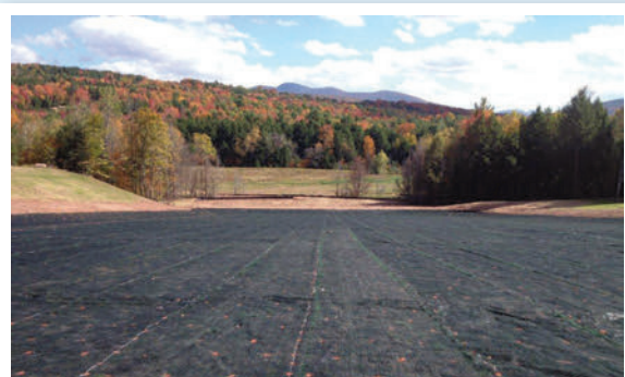
North American Green P550 turf reinforcement matting in place.
