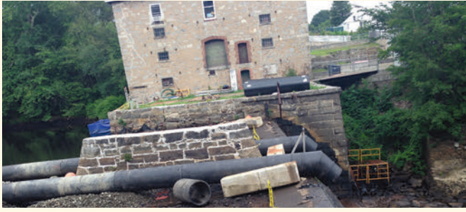
Sections of Snap-Tite rest beside the powerhouse, waiting to be installed from the upstream (left) side of the photo and exiting over the staging on the right side of the photo. Note the discharge piping in the foreground.
