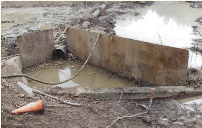
Long Creek Dirty Water
