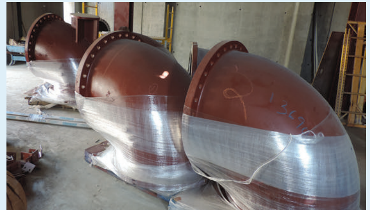
36"-diameter elbows supplied by Team QWP, waiting for installation.
