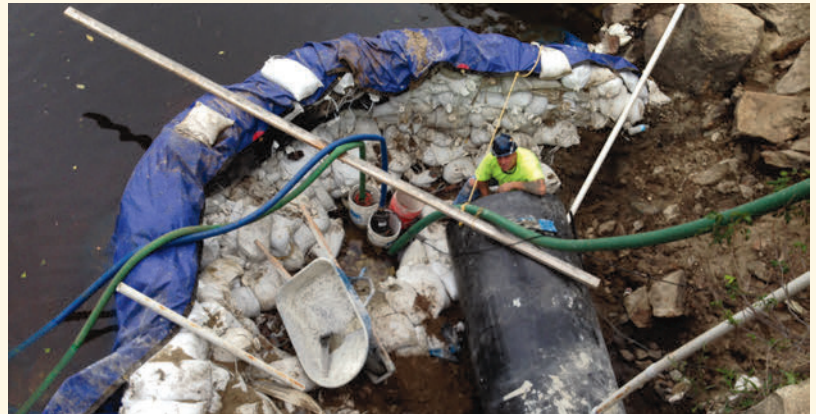
An R.T. Nunes employee monitors the inside of the Snap-Tite pipe while Team PPF grouts the annular space between the new and old pipes.
