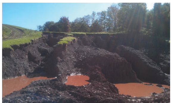
Devastated spillway caused by Hurricane Irene
