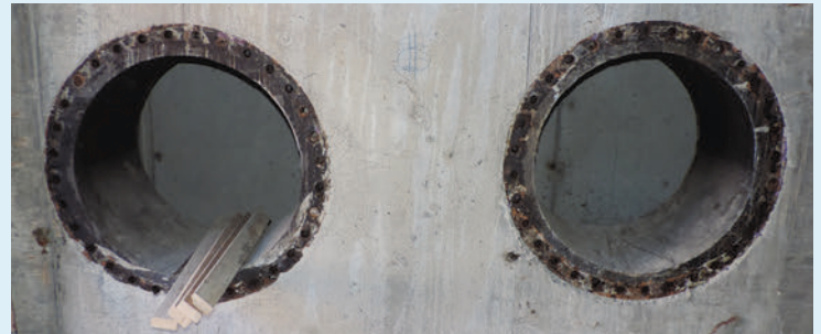
36"-diameter wall pipes cast in place in the new concrete structure.
