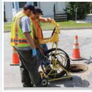
Town of Mexico, ME, and Team PPF with a 400-foot Pearpoint push camera inspecting 286 feet of 8-inch sanitary sewer pipe.
