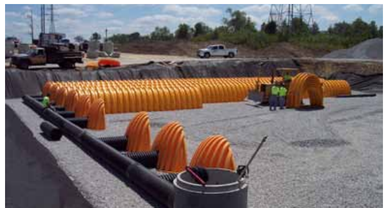
Earth Construction of Ft. Wayne, IN, is shown preparing the site for the installation of the ADS MC4500 Storm Tech Unit along with a 60" Water Quality Unit (6040).
