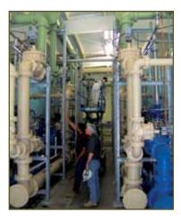
interrupting service. This meant developing and installing a bypass system capable of pumping 35 million gallons per day. The major improvements included installation of four 550 HP wet weather pumps, two 330 HP dry weather pumps, a 20,000 gallon surge tank (shown in the photo) and all associated large diameter valves and 36" and 42" process piping fabricated by Quality Water Products.
