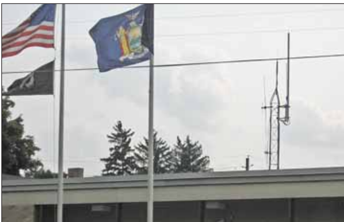
The FlexNet's advanced metering system does not require a separate tower structure; a FlexNet antenna can be placed on top of any building that is at least 37 feet tall. Shown here is the Tower Gateway Base Station antenna installed on top of the police station in Horseheads, NY. A special thank you for their role in installing the system goes to the principal players, Chris Lawrick and Sharron Cunningham, and Fred Kelley, Dick Kaulfuss and Josh Ordway from the "good guys" side.
