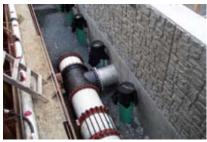
Pictured are some of the epoxy coated 48" fittings at the intake structure. During high tide, river water flows through the 48" and 36" pipelines so it can be treated.
