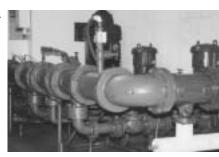
The existing steel pipe originally installed in 1993 was corroding and had started to form pinholes. EJP – Vernon contacted its sister company QWP and Jeff Carlos was sent to measure and lay out the project. The welded steel pipe with ductile iron flanged pipe and fittings were manufactured and shipped based on the dimensions he took at the site. The customer's comments say it all. *Great job, everyone.*
