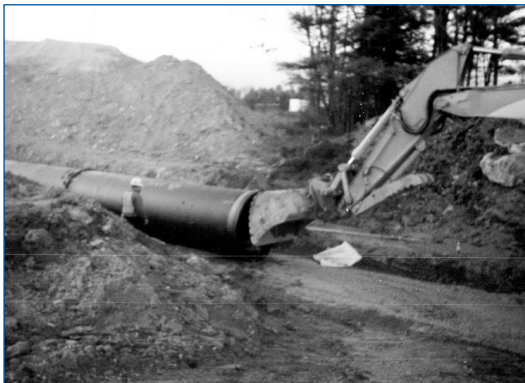
The Maine Turnpike Authority, R.J. Grondin, Woodward & Curran and Team EJP teamed up to reroute the 42" transmission main feeding the city of Portland from Sebago Lake.
