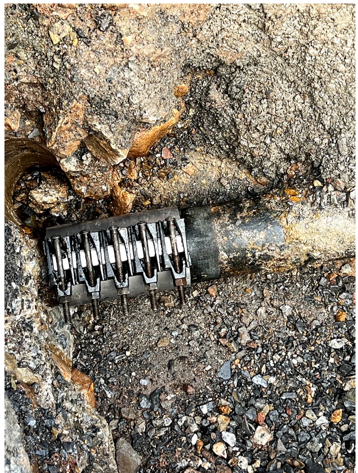
Photo of the repaired water line
